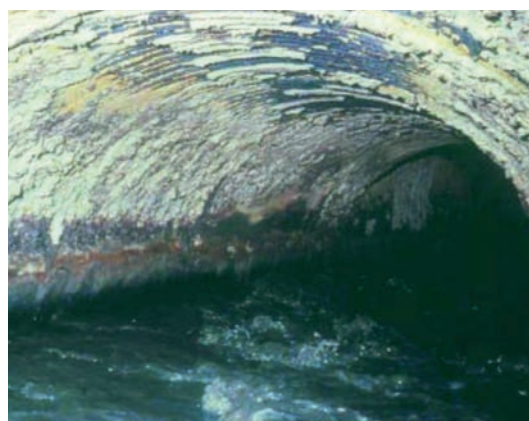
Effect of alkali-silica reaction (ASR) on a sewer
