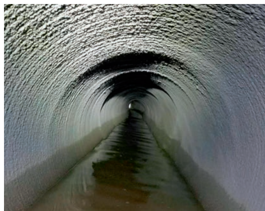
Sewer lined with BluCem ZeoGlass
