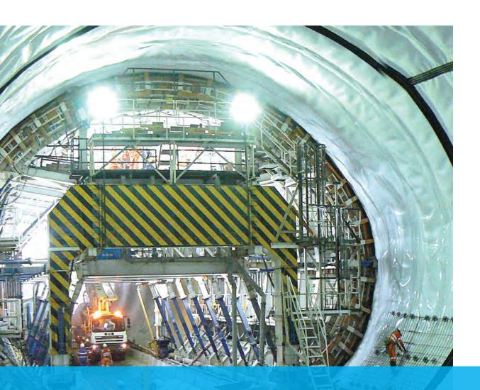
BluSeal Tunnel Liner ground water infiltration management
