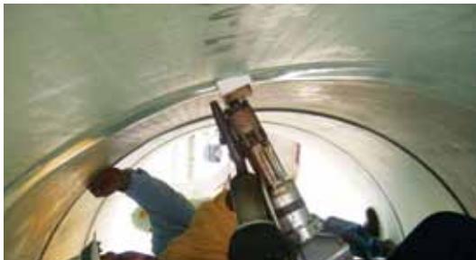
AUTOMATED PIPE WELDING ROBOT
