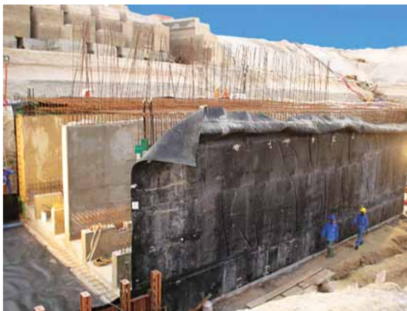
TUNNEL WATERPROOFING
