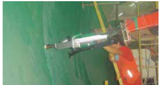
EXTRUSION SEAM SHOE CLOSE UP
